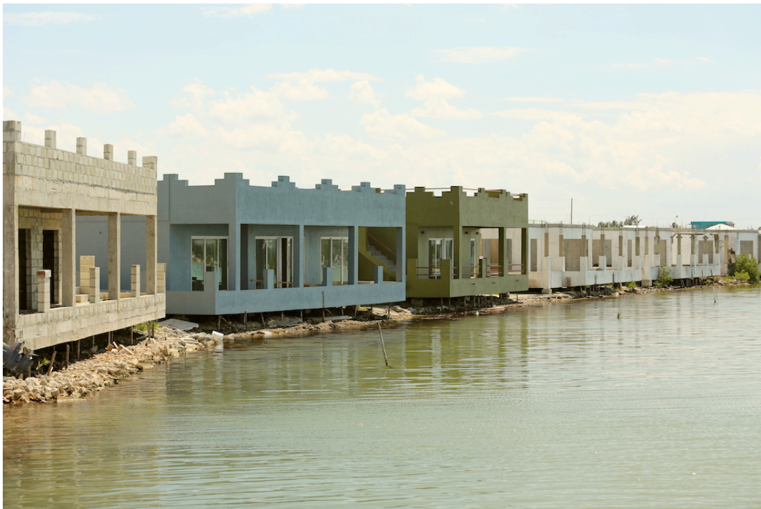
Figure 11 New housing development straddling water in Ambergris Caye Photo courtesy Sérgio Teixeira Santos
