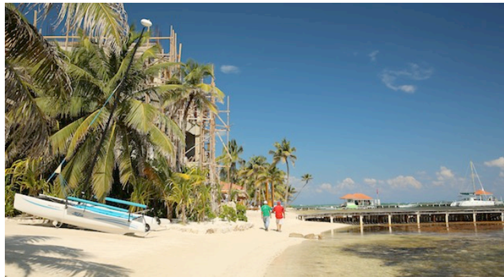
Figure 9 Resort in San Pedro, still in construction, straddling the coastline Leaves little more than one metre between the high water tide mark and the infrastructure limit.
